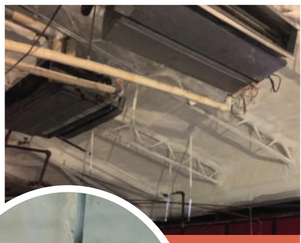
Different sections of the roof after the spray polyurethane foam application
