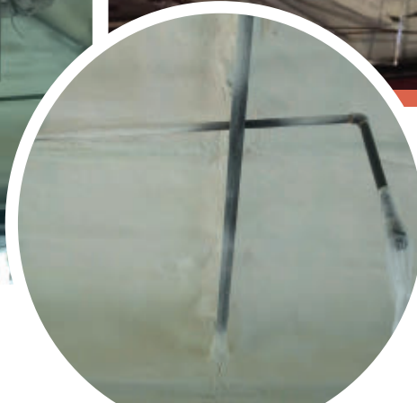
Different sections of the roof after the spray polyurethane foam application
