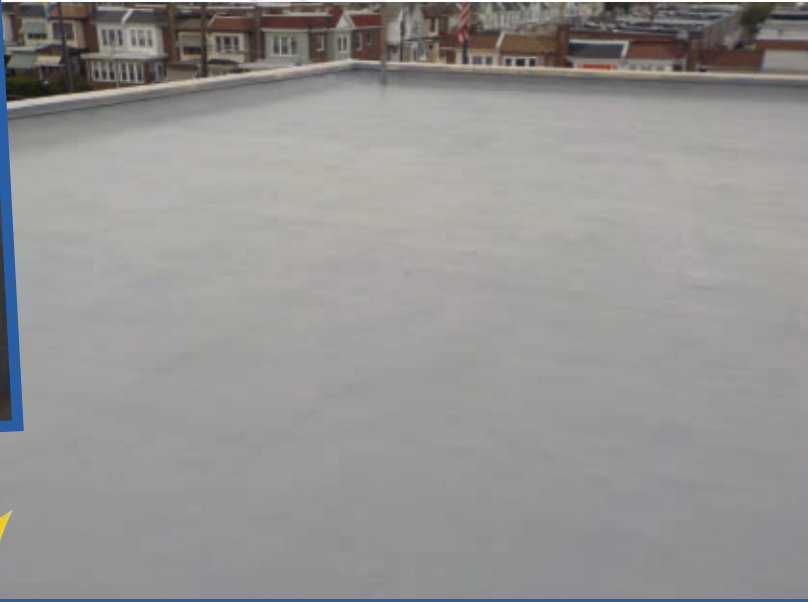
View of the roof after the grey silicone coating application
