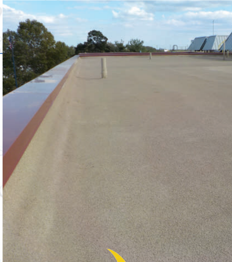
A tan, silicone coating was utilized for the topcoat
