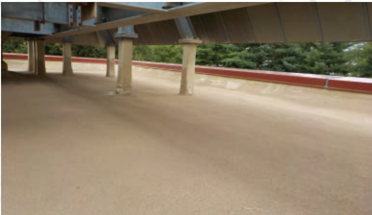
A tan, silicone coating was utilized for the topcoat
