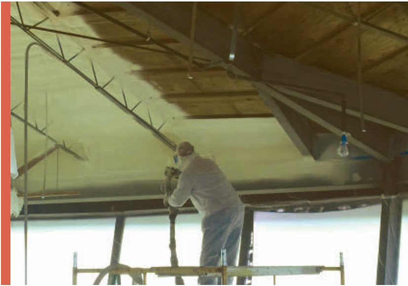
Purefoam Insulation applied closed-cell spray polyurethane foam to the underside of the roof
